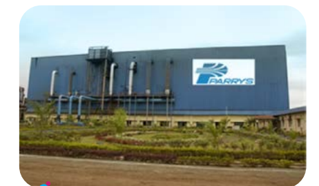
Integrated Sugar Factory consisting Sugar, Co-generation and Distillery Haliyal – Karnataka
