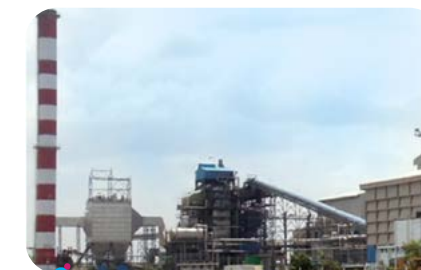
Integrated Sugar Factory consisting Sugar, Co-generation and Distillery Bagalkot – Karnataka
