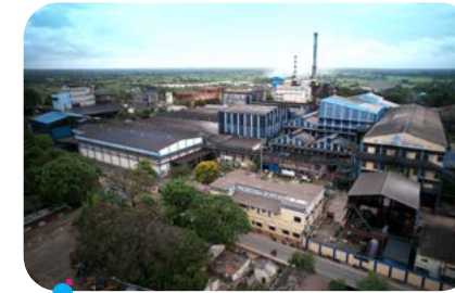
Integrated Sugar Factory consisting Sugar, Co-generation and Distillery Nellikuppam – Tamil Nadu
