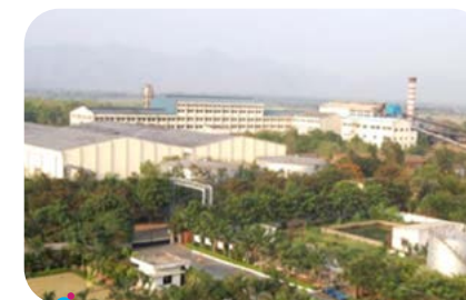
Integrated Sugar Factory consisting Sugar, Co-generation and Distillery Sankili – Andhra Pradesh
